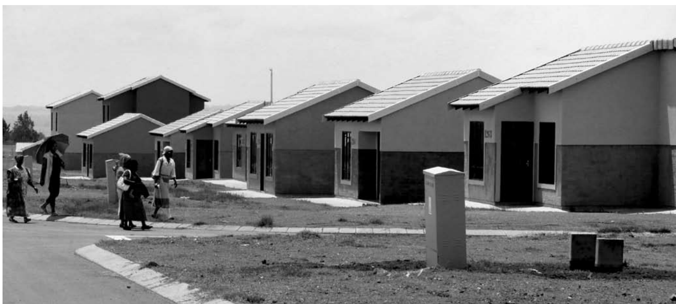
Delivery: Some of the 3-million subsidised houses built since the defeat of apartheid
